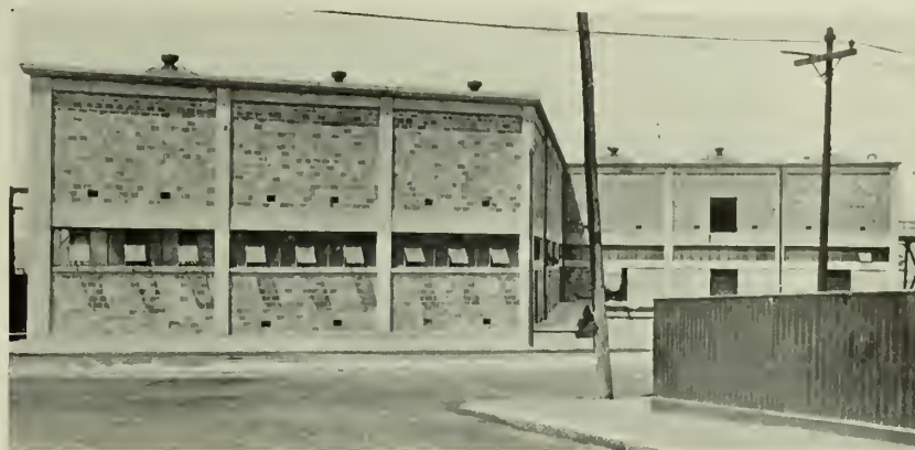
BUILDING FOR STANDARD OIL COMPANY, EAST BOSTON, MASS. Showing terra cotta hollow tile wall construction.
